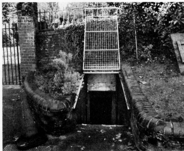
Entrance to the Boys' shelter - Photo by Bob Clary
